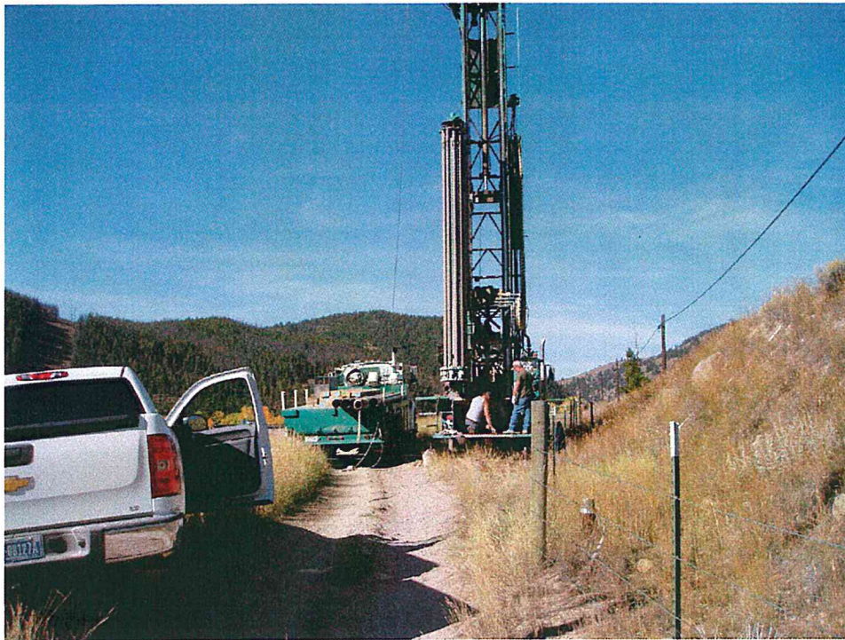
West well installation. Old well to the right of wooden fence post.
